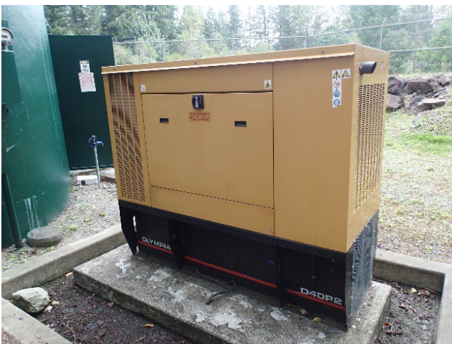
Lift Station Emergency Generator
